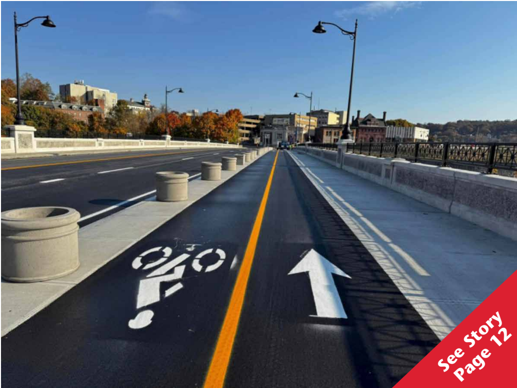
The recently completed Derby/Shelton Bridge enhancements.
